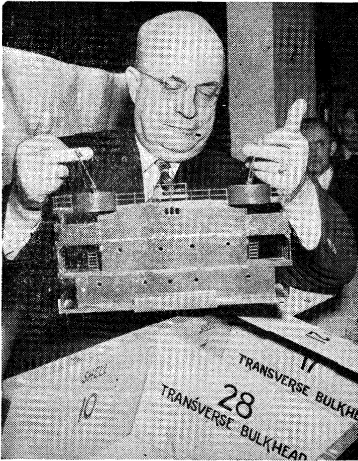
Henry J. Kaiser, U.S. shipbuilder and holder of the world records for building 10,500-ton Elbert cargo ships, demonstrates on a 14-foot demonstration, he put together the prefabricated, numbered parts in 7 minutes in the same way his shipyards assemble sections and launch model how his mass prefabrication production system works. In this the vessels in a few days.
